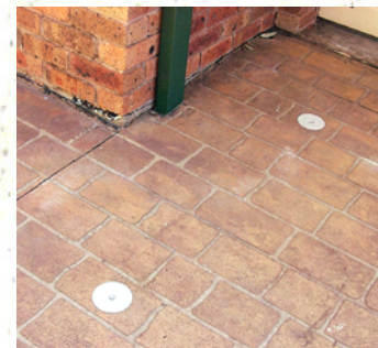
Installation through concrete.
