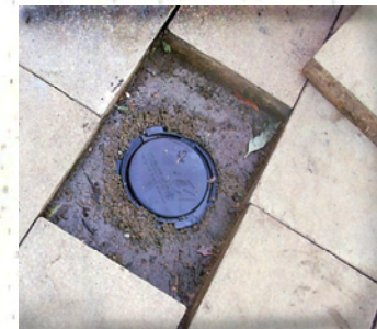
Installation under pavers
