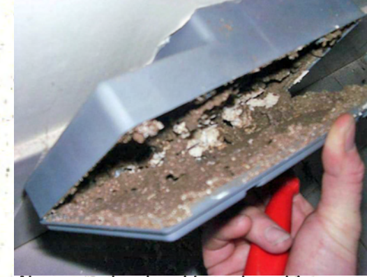
Above ground station with termite activity.
